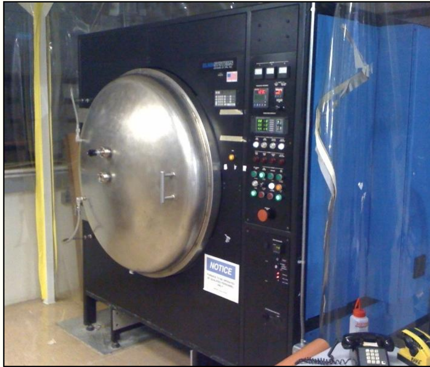
Jefferson Lab oven presently used for hydrogen degassing of all Americas Region cavities
